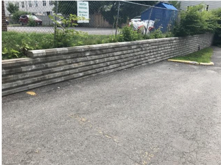
Retaining Walls Retaining Walls
