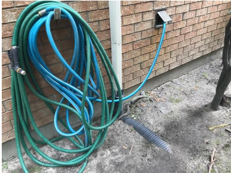
Soffit, Fascia, Gutters & Downspouts
