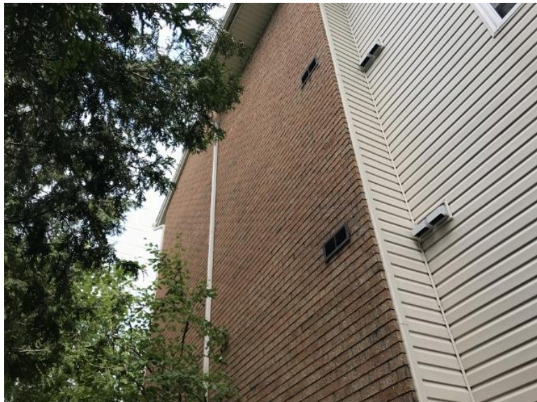
Exterior Walls Exterior Walls
