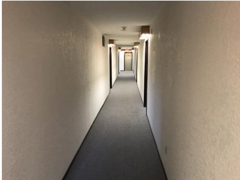
Interior Walls Interior Walls
