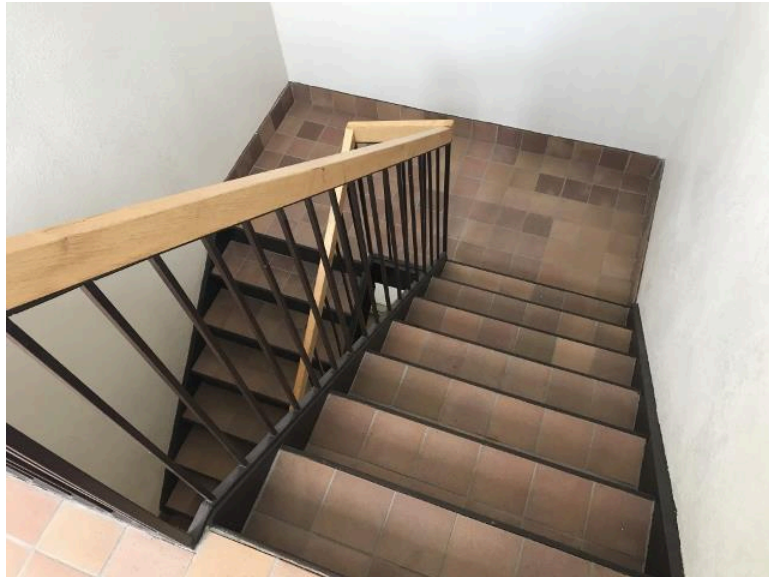
Stairs, Guards and Handrails Stairs, Guards and Handrails
