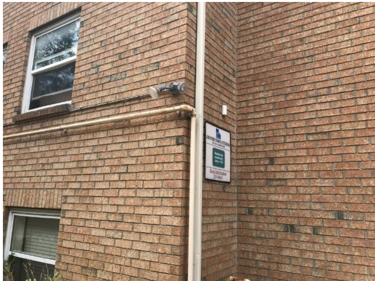
Area and Security Lighting Area and Security Lighting
