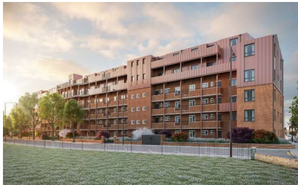
Two Storey roof top extension UK social housing program using modular components
